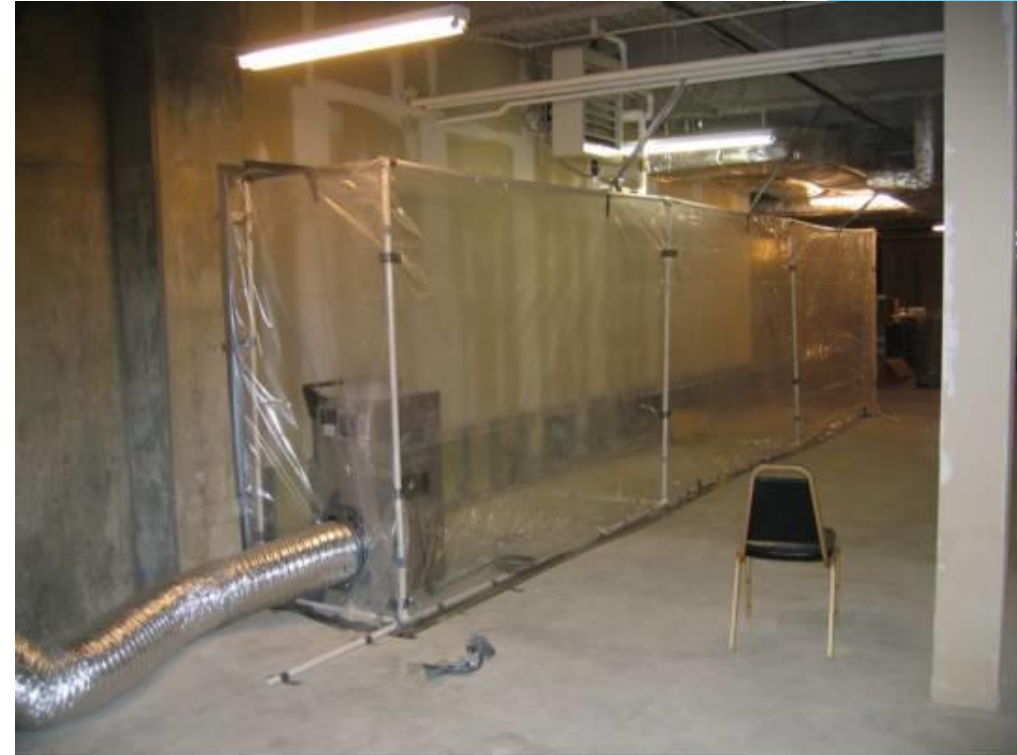
Mold Containment with Negative Air HEPA Filtering
